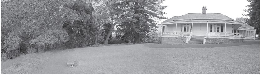
Figure 1. View of House and garden looking south east (courtesy Hamish Macdonald).
